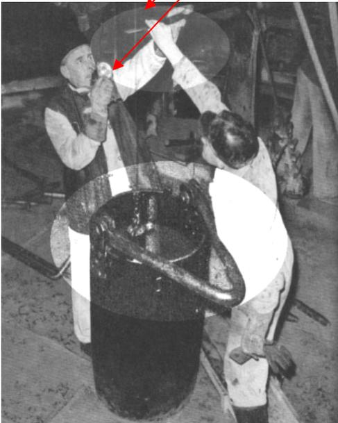
2 PLUMB BOBS IN A WATER BUCKET (to reduce the oscillation)
