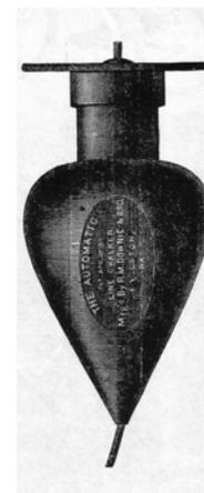
C 4 d) In this decorative example, a recoiling string mechanism is applied to an internal reel, thus the line is retracted into the chalk reservoir.
